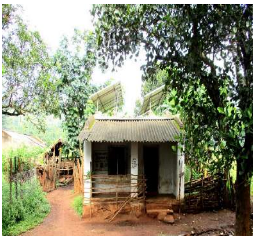
The solar-powered millet processing unit at Dupi
