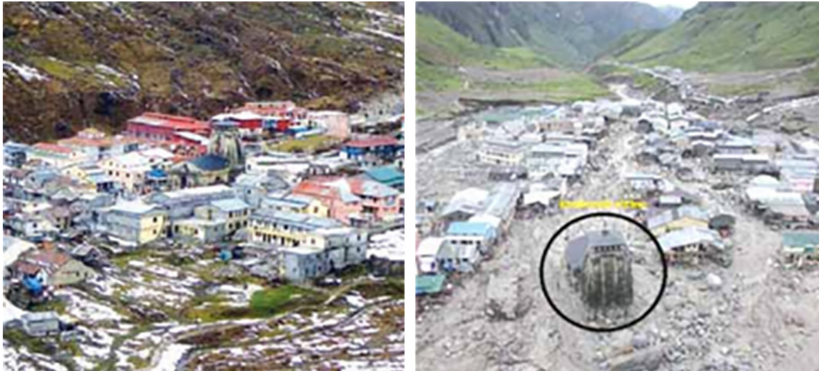
Figure 7: Kedarnath Before and After the Flood
