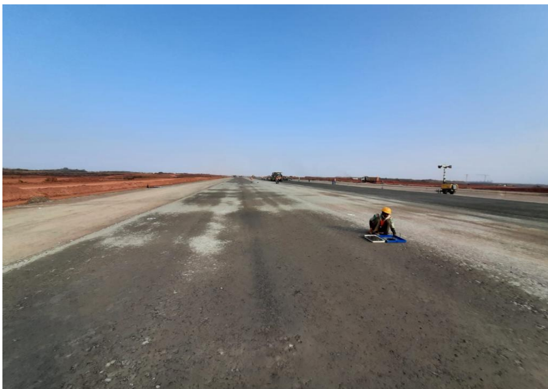
Figure 30: Runway Earthworks at Mopa Airport Project Site
